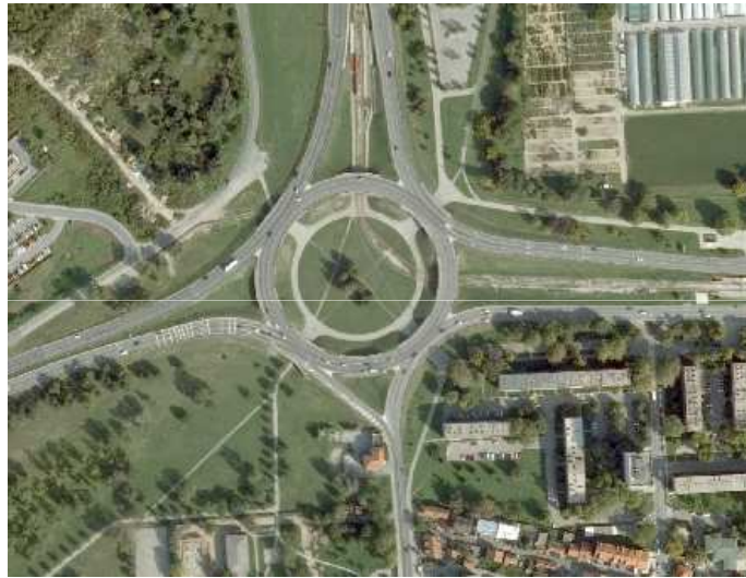
Figure 2. Big roundabout ( D_v = 148 m, n = 3/3 ) Jadr. Ave. – Remet. Str. at entrance in Zagreb, 1980.
