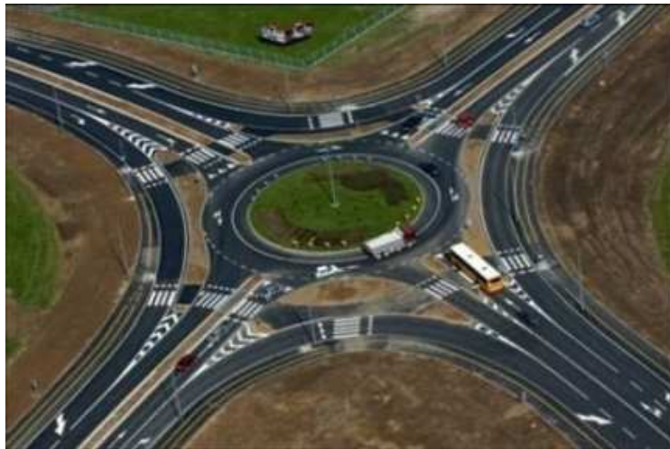
Figure 6. Direct weaving of cars, bicyclists and pedestrians by independent guiding (Varaždin bypass, 2005)
